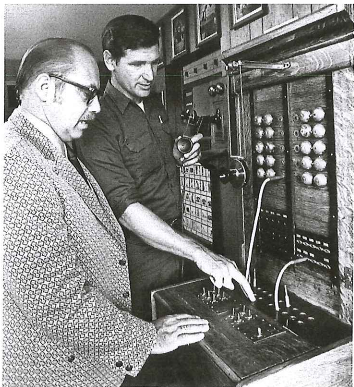
John Murphy, president of the Gorham Telephone Company, explains the operation of an 1890 R&R electric switchboard to Ehly.
